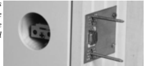
Figure 27: Screws should connect the deadbolt plate to the stud
