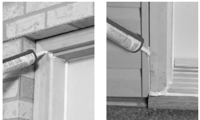
Figures 31 and 32: Caulk the jambs and the exterior trim.
