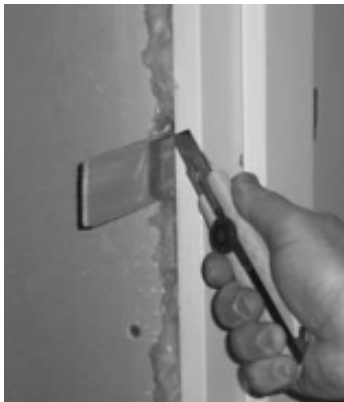
Figure 28: Score and snap shims.
